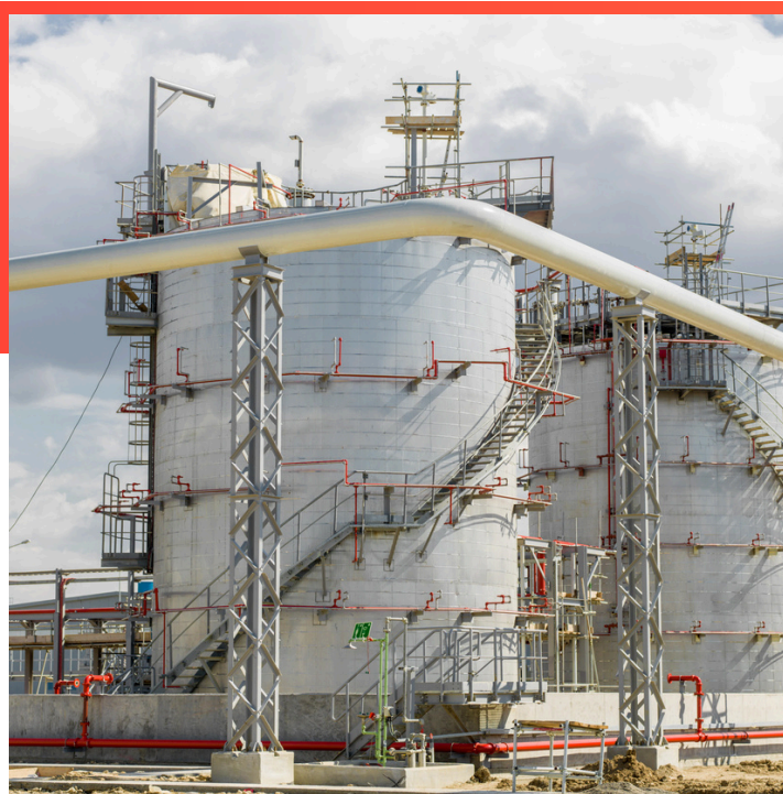
Oil & gas piping construction
