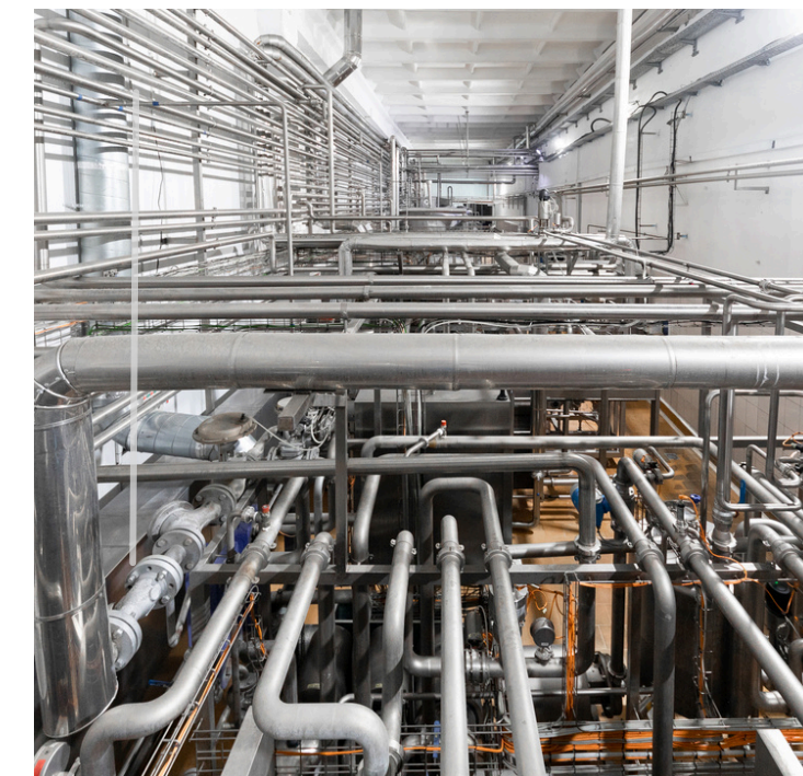
Plant piping construction
