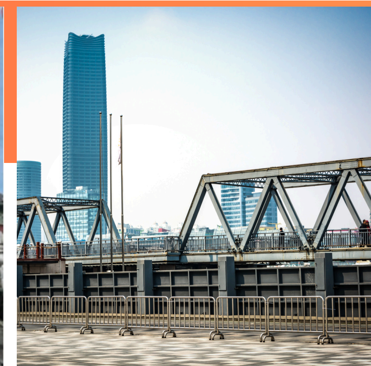
Steel structure construction
