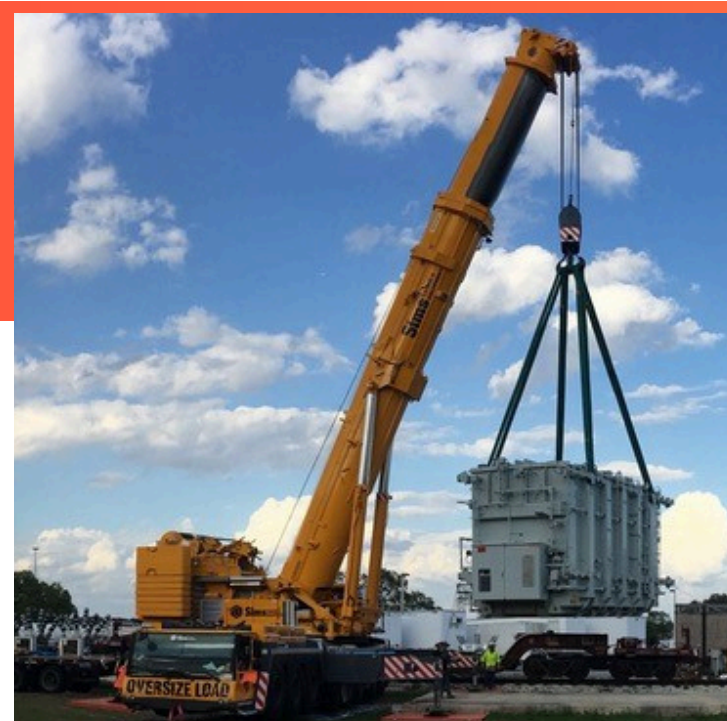
Transformer erection
