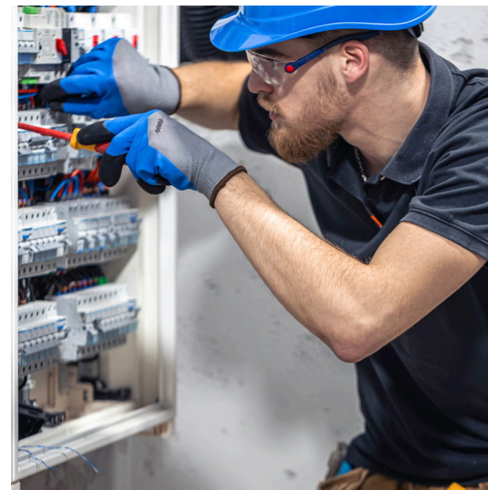
Electrical panel wiring
